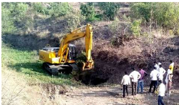
Canal deepening/desiltation
